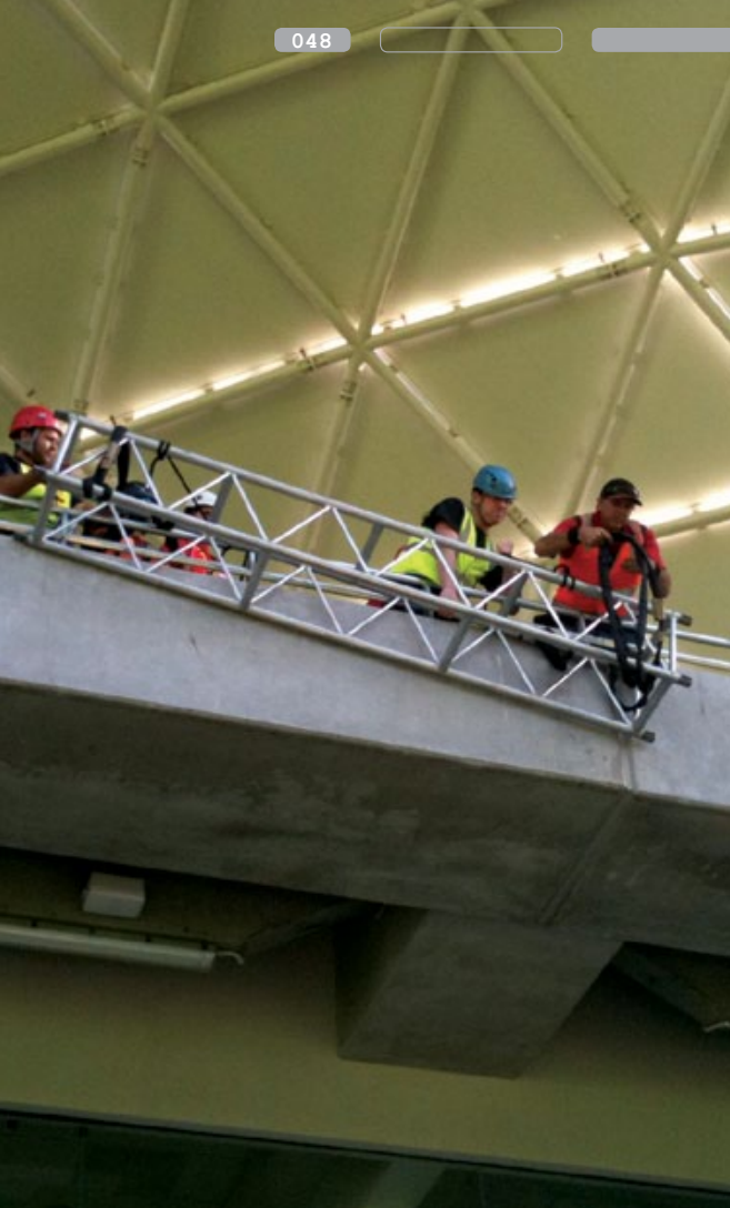
Roundslings and acres of burlap padding were required to suspend the 256m of lighting truss from the front of the east and west balconies.
