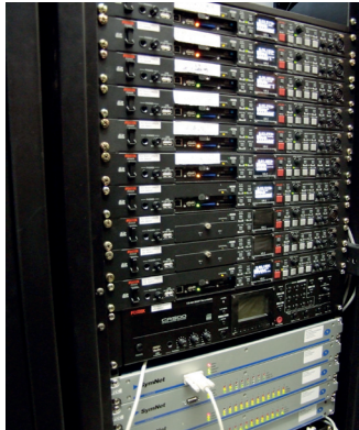
Racked Fostex UR2 stereo memory recorders, Symnet Express processors and Furman power conditioners
